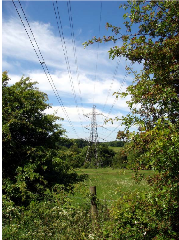
Photo 1 - Sample Caption - Power lines near sample customer
